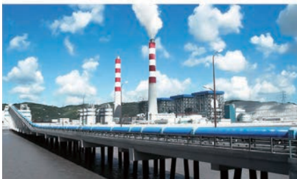
SAIF 225MW Gas Turbine Combined Cycle Power Project, Pakistan
