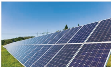
Yuzhou Peak Photovoltaic Power Station Project
